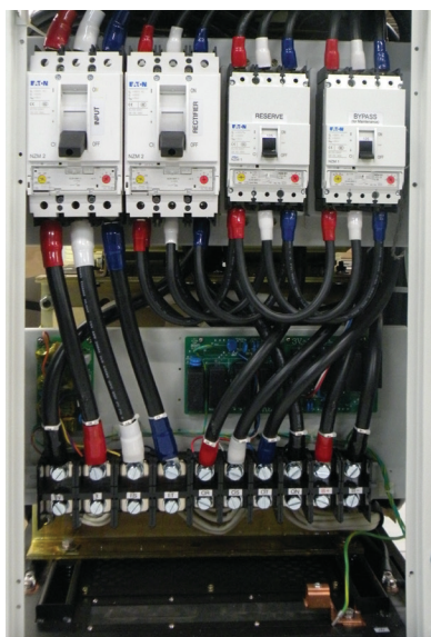
Standard Bottom Access Plate and Terminal Block Connections
